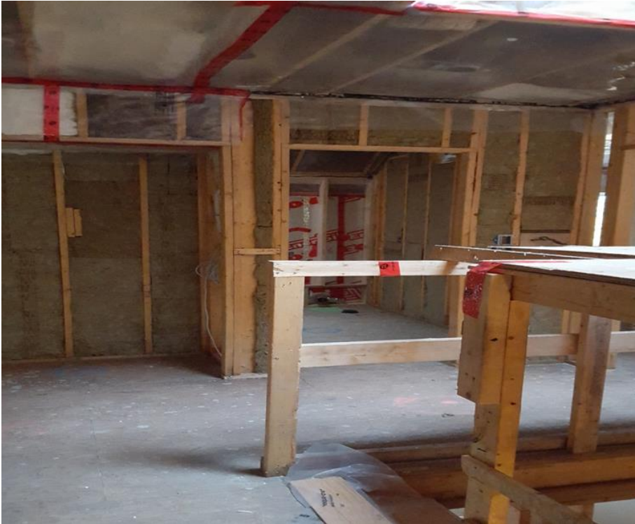
Properly sealed Attic
