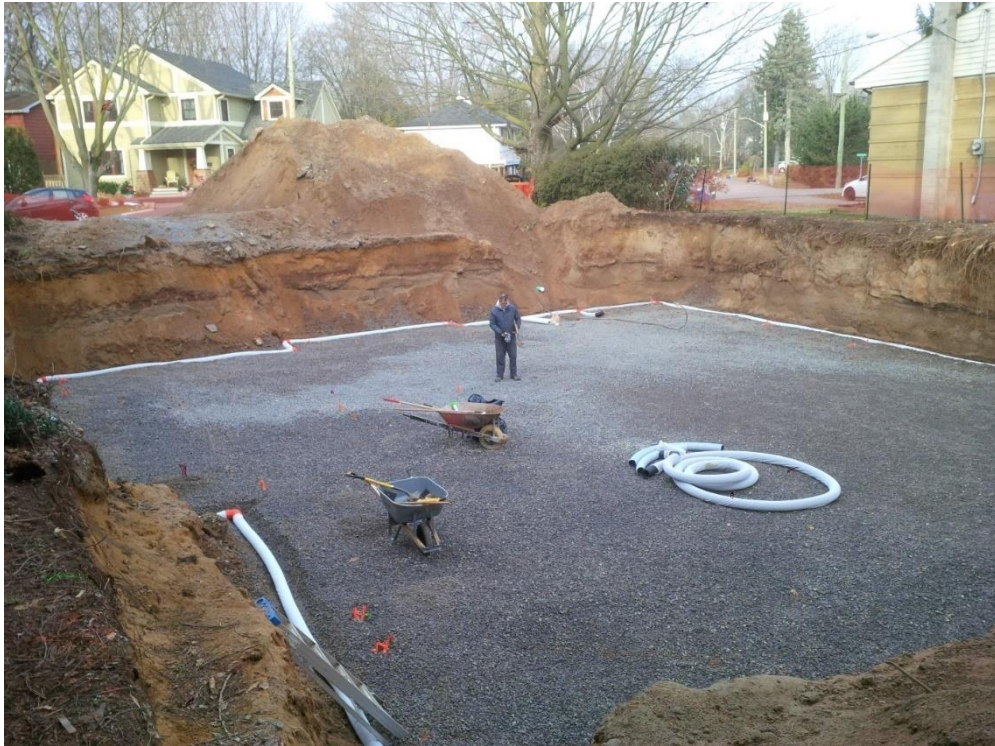
Clean and organized construction site
